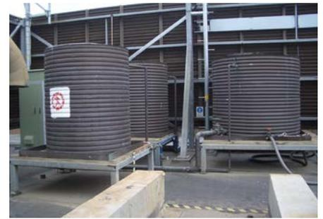
Figure 3: Flusher header tanks
