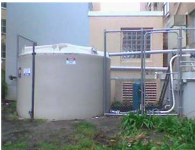
Steriliser water reclaim tank
