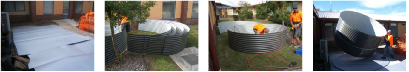
Figure 1: Installation of site built tank in internal courtyard
