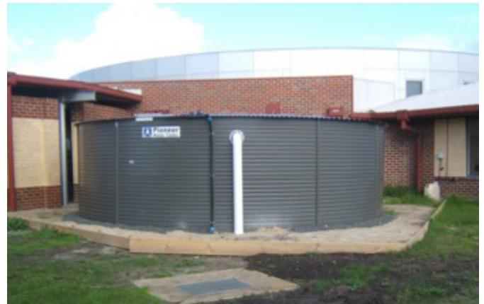
Figure 2: 95,000-litre site-erected tank
