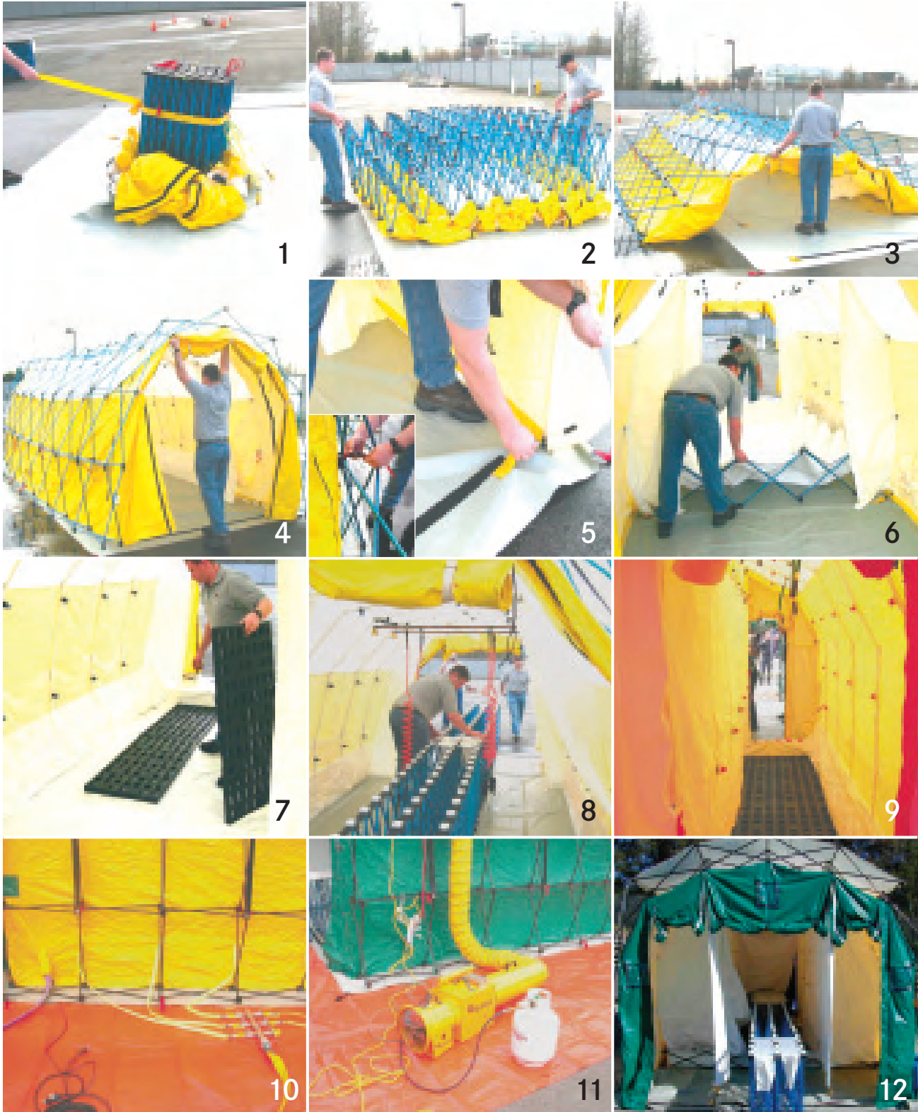
1-5. Deployment and raising shelter structure.
