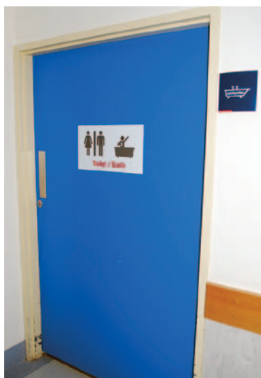
Doors accessed by patients are in a contrasting colour to walls
